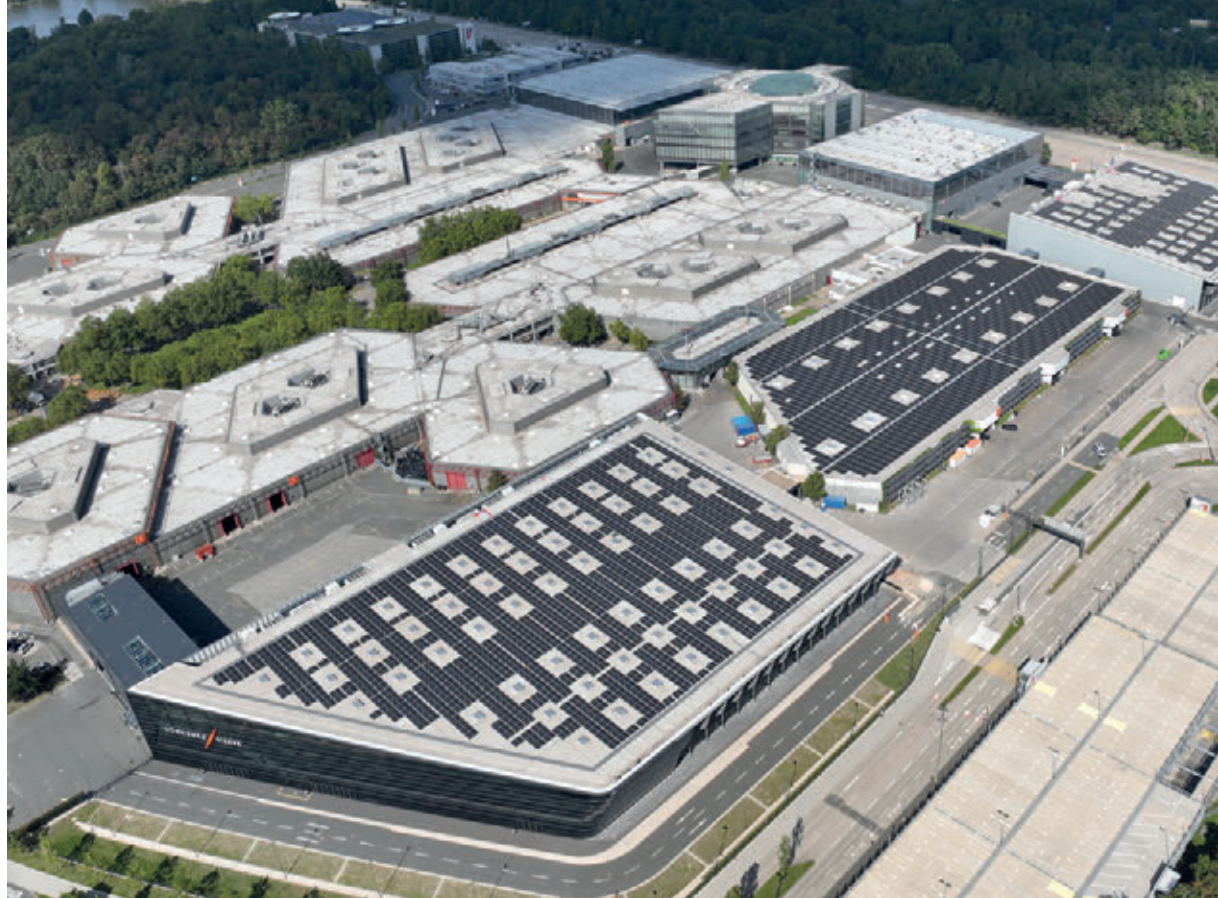
The Exhibition Centre draws 100 percent solar electricity from the photovoltaic system on its roofs.
